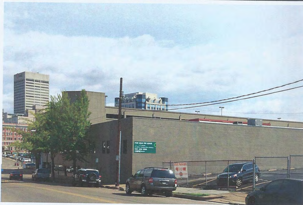
existing building for demolition
